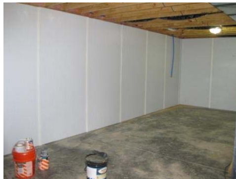
Fire rated insulation in basement
