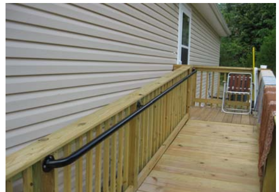
Handrail along ramp
