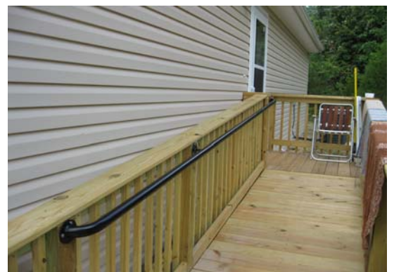
Handrail along ramp
