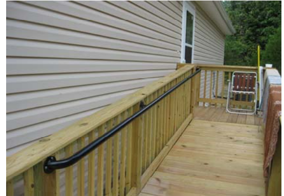
Handrail along ramp
