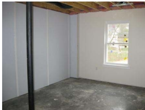
Fire rated insulation in basement
