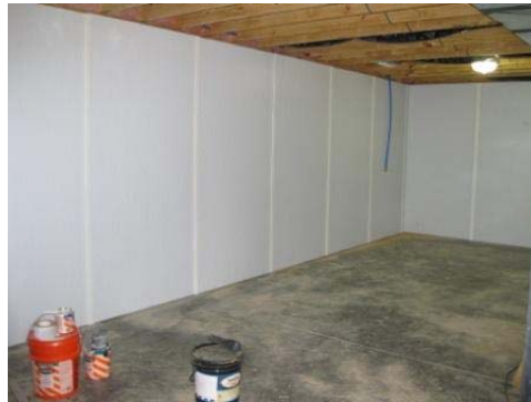
Fire rated insulation in basement
